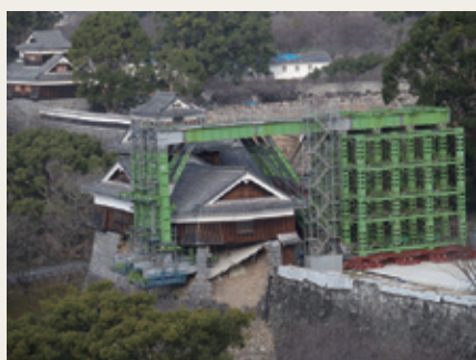
▶修復作業が進む熊本城
